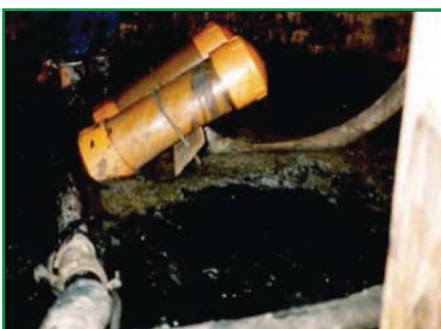
Before HydroLock Degassing and Cleaning
